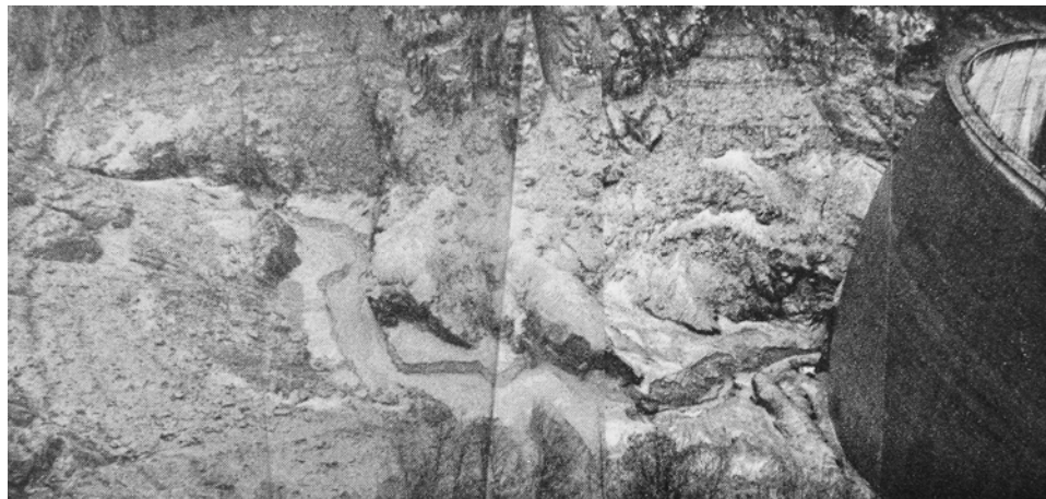
FIGURE 21.5 General view of reservoir upstream of Gebidem dam in 1995, after 27 years of operation with annual flushing ( G. Morris ).
