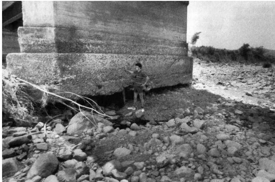
FIGURE 18.5 Streambed degradation and resultant bridge scour about 2.5 km below Patillas Dam, Puerto Rico ( G. Morris ).
