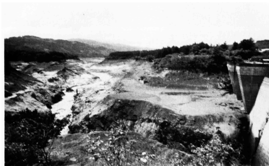
FIGURE 19.3 Photograph of empty Cachí reservoir during flushing looking upstream from the dam, showing channel and river terrace near the dam (G. Morris).
