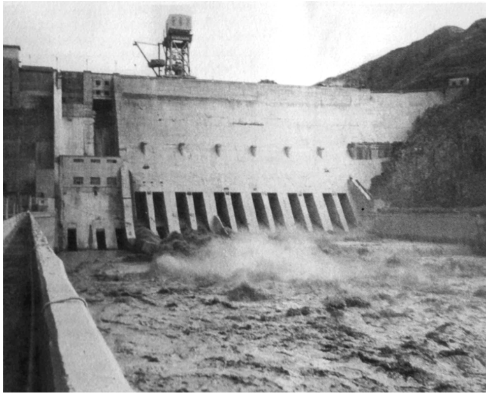
FIGURE 24.4 (b) Downstream face of Sanmenxia Dam during sediment flushing showing flow exiting from the sediment sluices (G. Morris).
