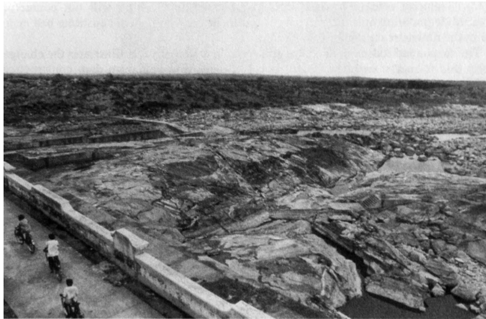
Figure 18.4. Photograph of area of scoured bedrock immediately downstream of Nizam Sagar Dam, Andhra Pradesh, India (G.Morris).
