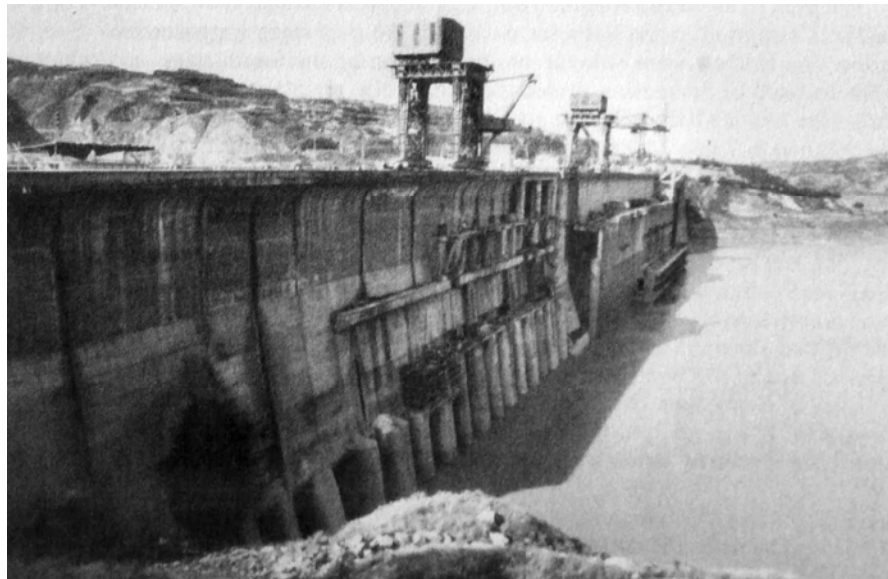
FIGURE 24.4 (a) Upstream face of Sanmenxia Dam during sediment flushing, showing low pool and low level sluices in the foreground ( G. Morris ).
