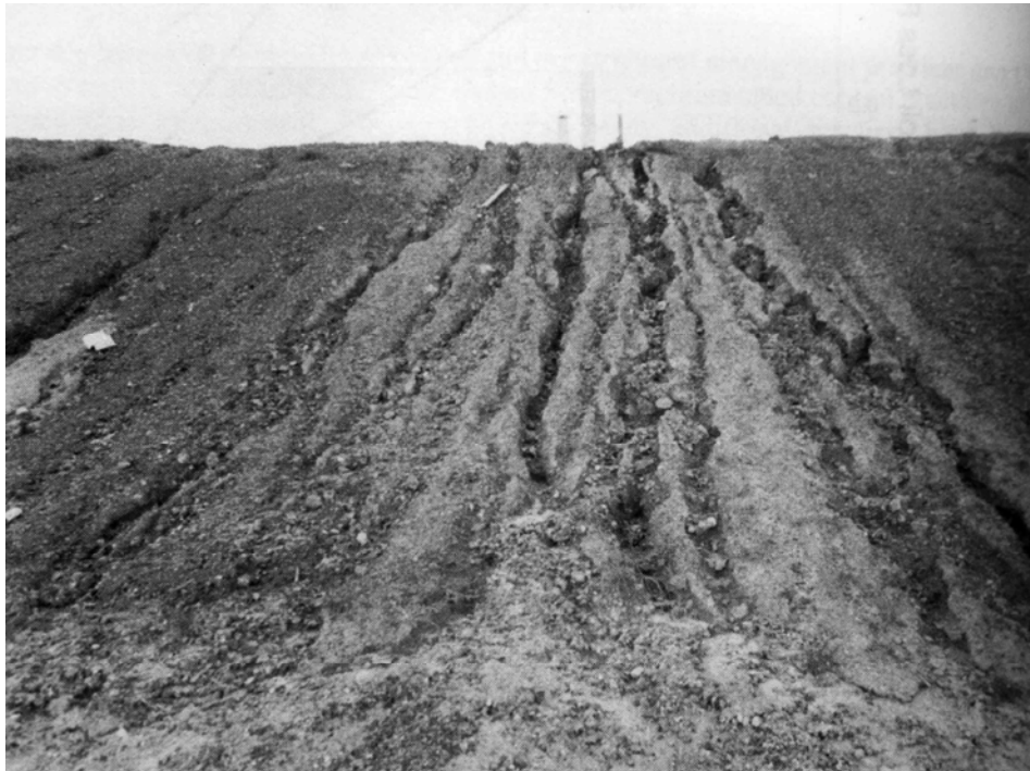
FIGURE 12.3 Concentrated runoff released downslope produces rill and channel erosion. Avoid this type of erosion by diverting flows away from unprotected slopes and providing protection where the flow is released downslope ( G. Morris ).
