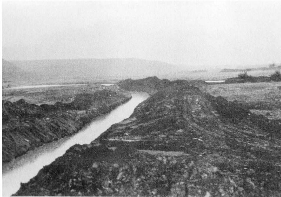
FIGURE 23.18 Photograph of upper reach of pilot diversion channel prior to erosion ( E. Tolouie ).
