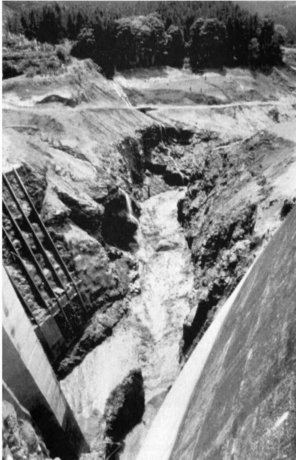
FIGURE 19.6 View from the darn during flushing looking down on the flushing channel and power intake at Cachí reservoir. The intake is located adjacent to the thalweg in an area affected by turbidity currents. This location facilitates sediment removal from in front of the intake during flushing, as shown ( G. Morris ).
