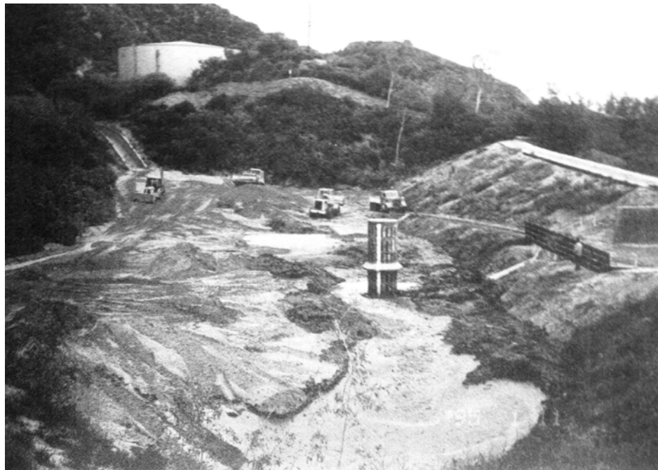
FIGURE 12.25 Cleanout of a debris basin operated by Los Angeles County, California. Note the perforated riser for drainage of the basin ( M. Bolander ).
