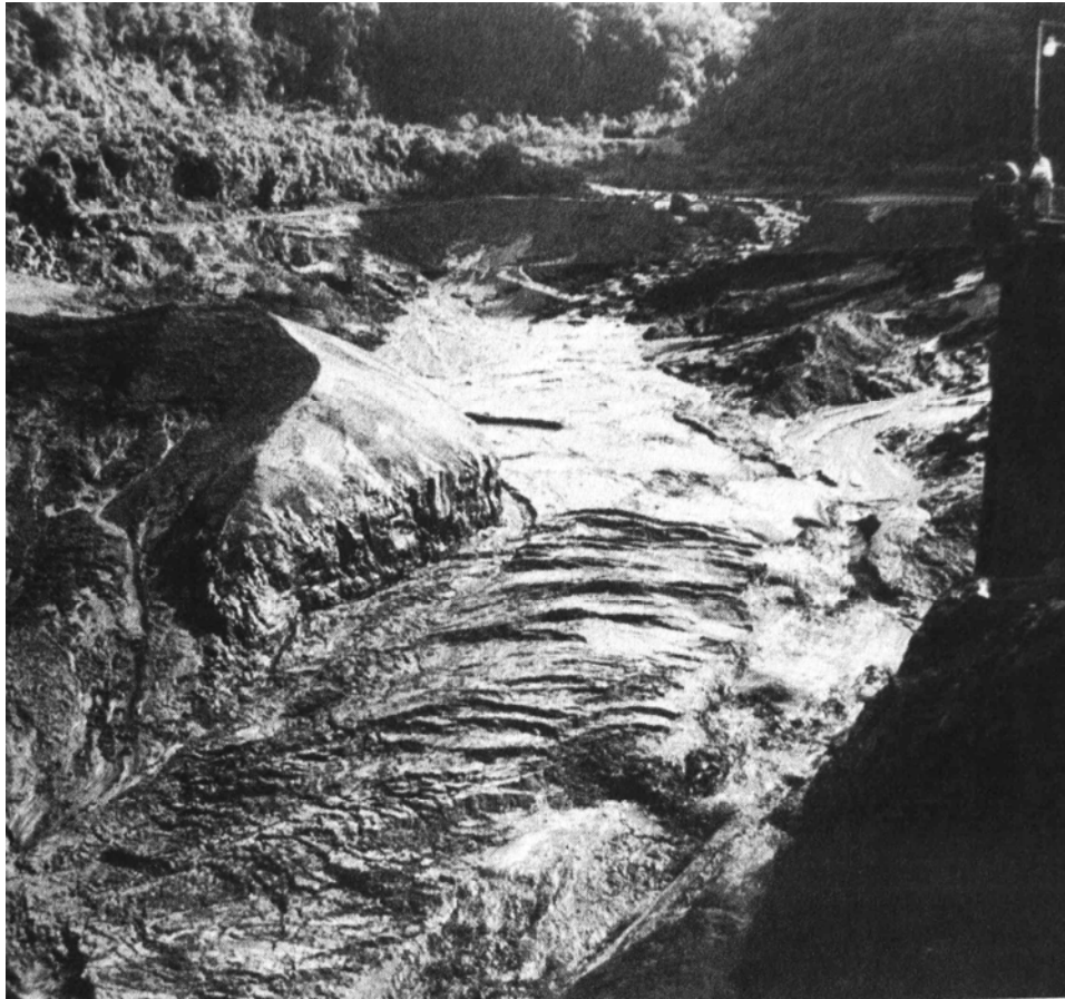
FIGURE 15.11 Slumping of fine-grained deposits near the dam in the small 285,000 m 3 Santa Maria reservoir on Río Samala, Guatemala, as sediment is discharged through bottom outlets. Sediment slumping was accelerated and removal enhanced by closing gates to temporarily inundate the deposits, then draining the reservoir a second time (V. Galay).
