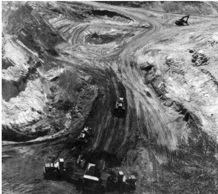
FIGURE 16.1 Photograph of sediment removal at Cogswell Reservoir ( courtesy Los Angeles County ).
