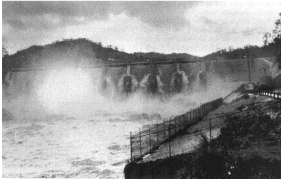
FIGURE 20.2 Overtopping of Loíza Dam during hurricane Hugo, 1989 (G. Morris).
