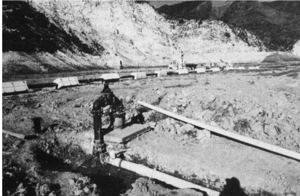
FIGURE 13.13 Well drilled into empty Gibraltar Reservoir, California, during drought. The photograph also shows dredging equipment left stranded by the drought ( G. Morris ).
