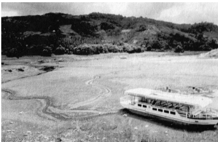
FIGURE 19.4 Photograph of left side of Cachí reservoir during flushing showing broad flat terrace. The main flushing channel is in the background at a lower level and is barely discernible ( G. Morris ).
